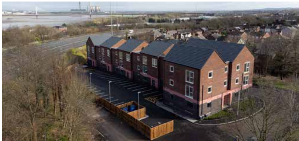
Sewell Street, Runcorn
